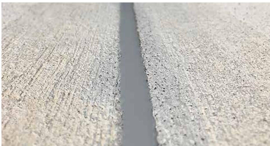
Querfuge Betonplatte, Kaltverguss PMMA
