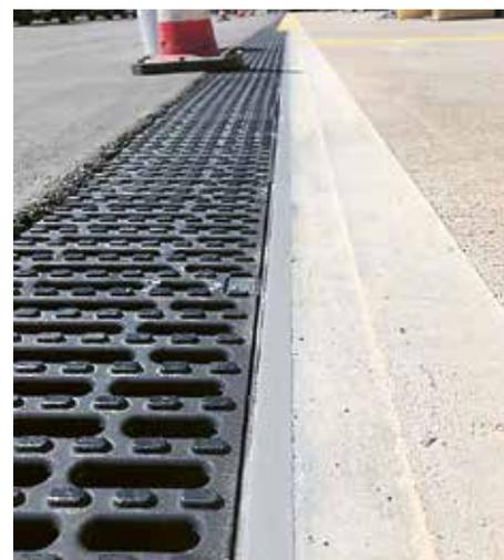
Fuge Betonrinne, Kaltverguss PMMA
